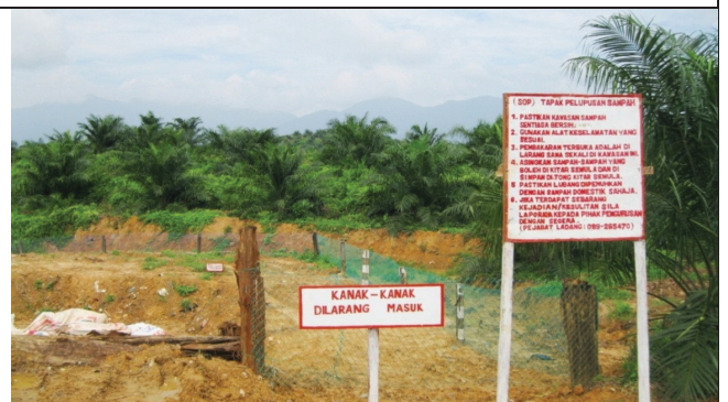
Maintenance of landfill site at Tangkulap estate.
